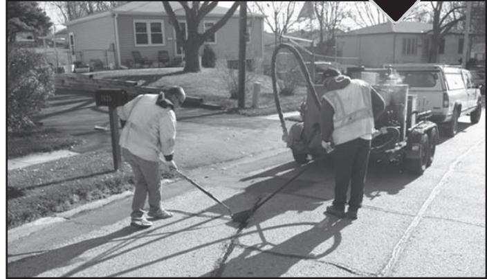
Public Works crews use a high volume, high pressure pull behind air compressor with a wand attached to the compressor hose to blow the cracks and joints clean and to dry them.
