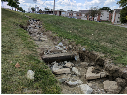
OPEN DRAINAGE CHANNEL WITH SEVERE EROSION
