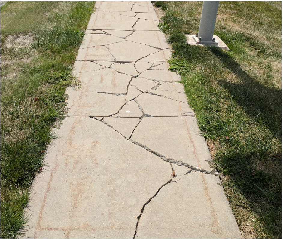
EXISTING 4' DETACHED SIDEWALK IN POOR CONDITION
