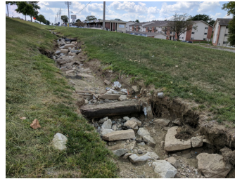
OPEN DRAINAGE CHANNEL WITH SEVERE EROSION
