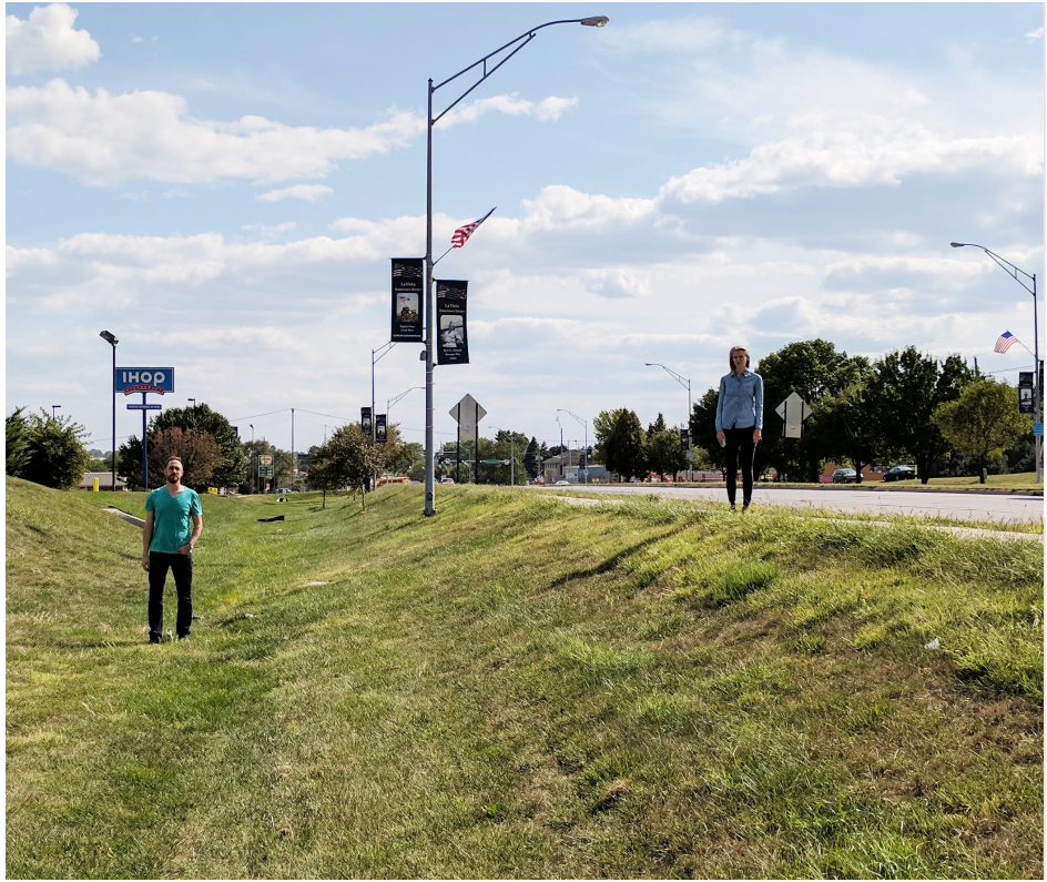
OPEN CHANNELS CONVEY STORMWATER AND ARE CONSIDERABLY LOWER THAN THE ROADWAY
