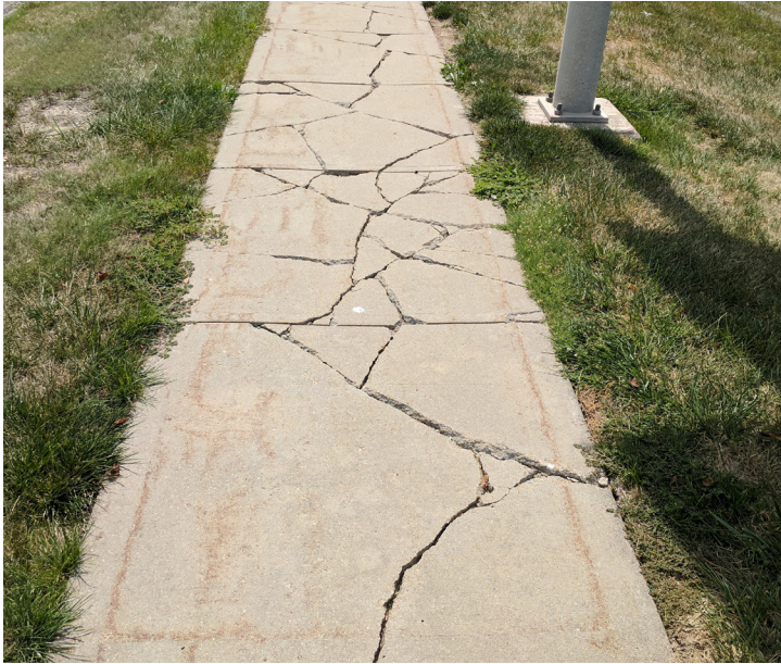
EXISTING 4' DETACHED SIDEWALK IN POOR CONDITION
