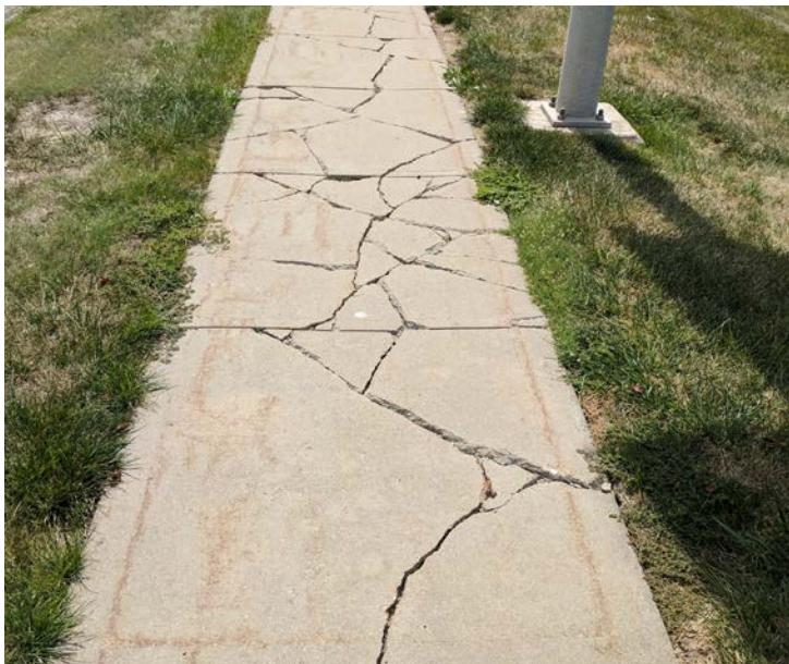
EXISTING 4' DETACHED SIDEWALK IN POOR CONDITION
