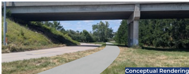
Eastport Parkway looking west (from bridge location)
