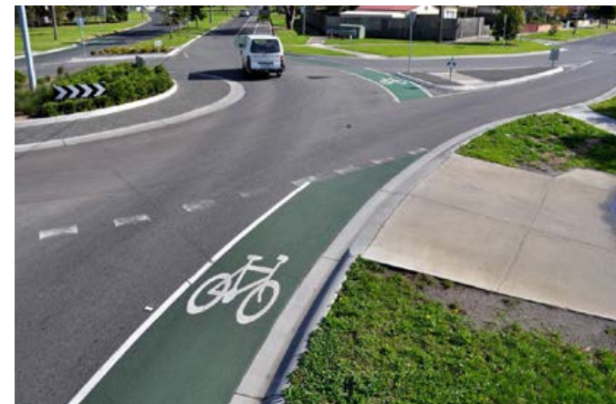
Bike lanes through a roundabout
