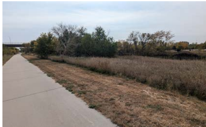
Bridge location looking southwest
