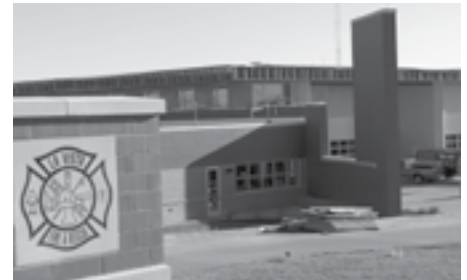
Fire Station No. 2 nearing completion.
